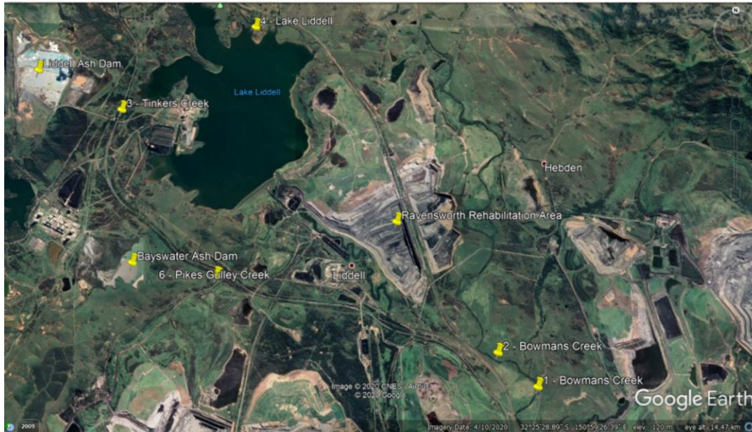
Figure 1: Central Hunter River Valley including Lake Liddell, Liddell and Bayswater Power Stations and ash dumps
