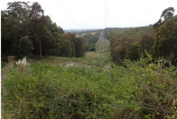
Plate 13. View to east. Cleared transmission easement after it deviates to the east. Looking down to gully of Maryland Creek.
