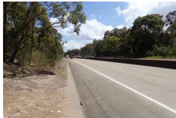
Plate 2. View to west. Newcastle Link Road (A15) follows a ridge crest, and runs through the centre of the study area from east to west. Road corridor is highly disturbed.
